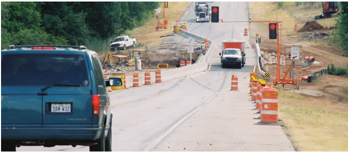
Use of portable traffic signals during construction
