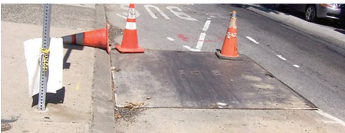
Use of steel plates during construction
