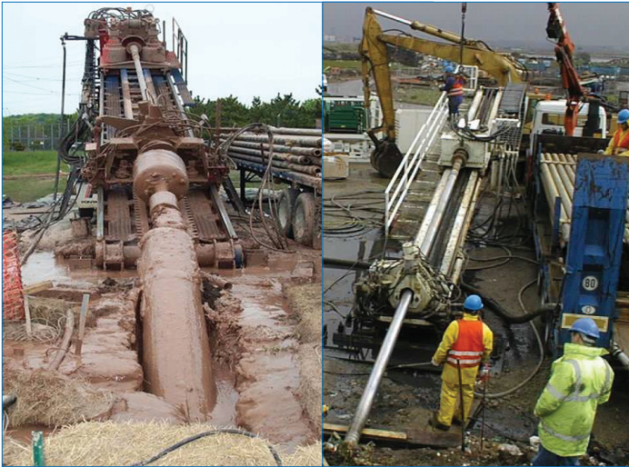
Typical horizontal directional drilling machines
