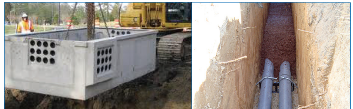
Common duct bank and manhole installation activities
