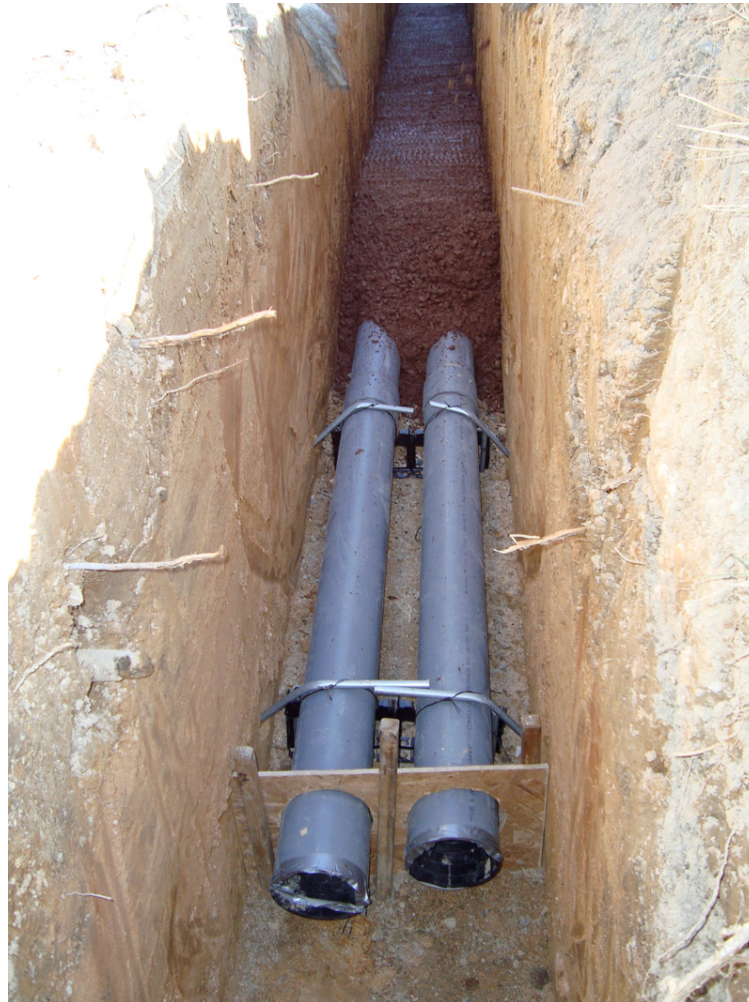
Example of Duct Bank Being Installed
